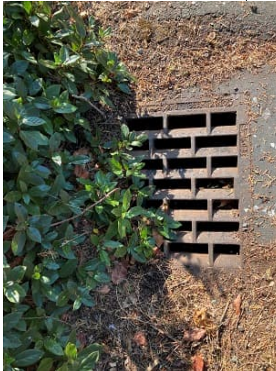
Picture 10 ROW in front of 3632 73 rd Avenue SE (south)
