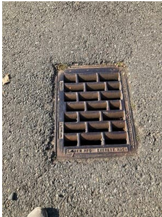
Picture 19 ROW in front of 3696 72 nd Place SE
