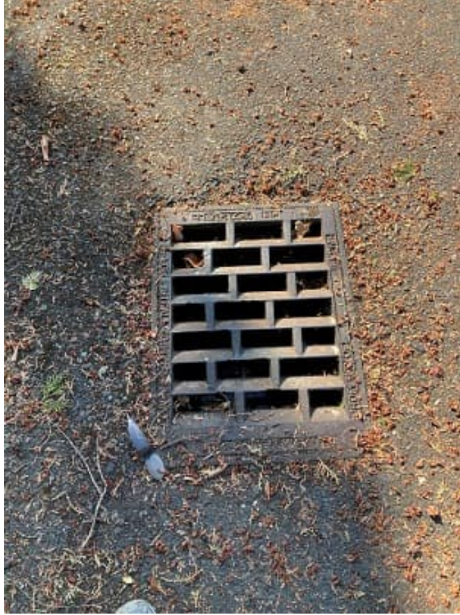
Picture 9 ROW in front of 3622/32 73 rd Avenue SE
