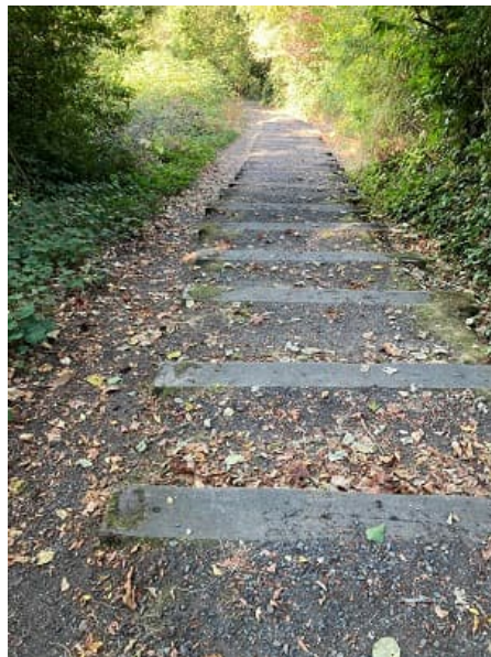
Picture 15: SE 38 th Street ROW Engineer could not locate the two catch basins in this area.
