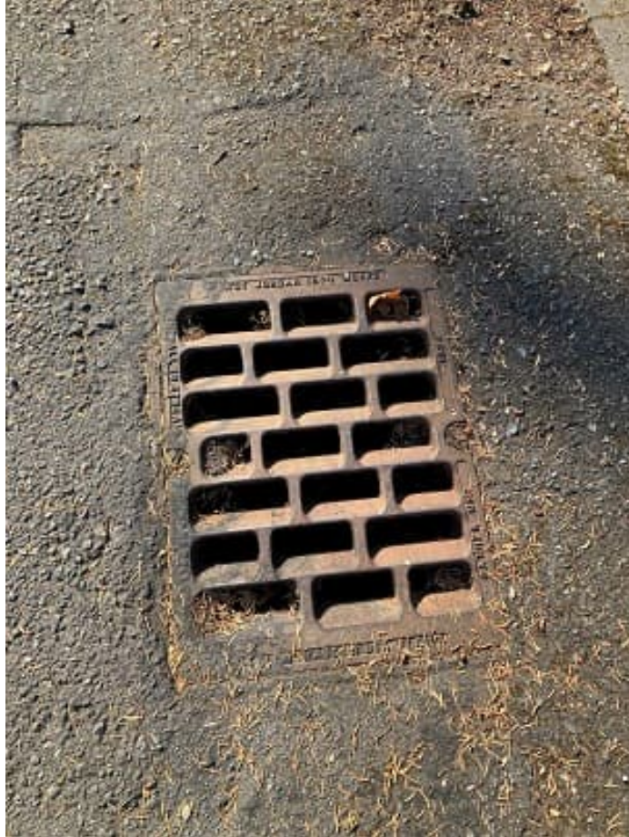
Picture 2 ROW in front of 3449 72 nd Place SE 8" DI pipe discharging toward the south leads to this catch basin.
